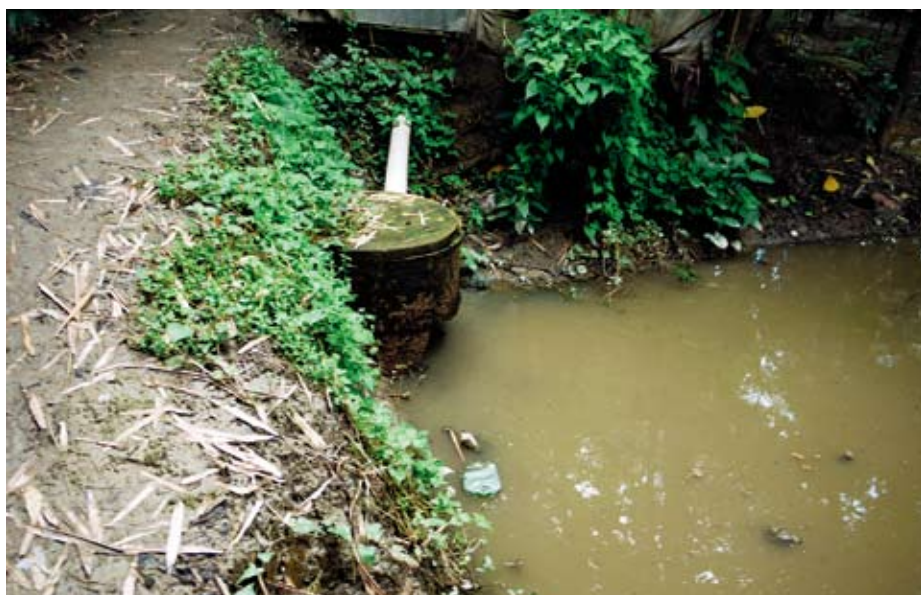
Figure 2 depicts a typical example of a failing latrine tank leaking into a pond.
